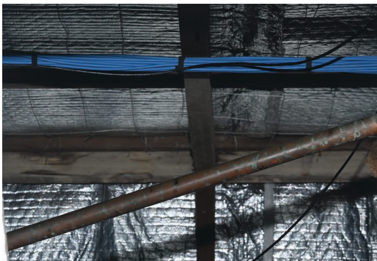
Photograph 9 Inspection of ceiling voids Paterson House
