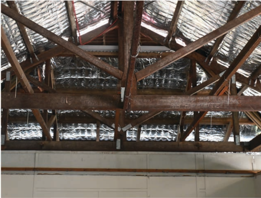
Photograph 6 Heritage Playshed Eastern Elevation Ceiling
