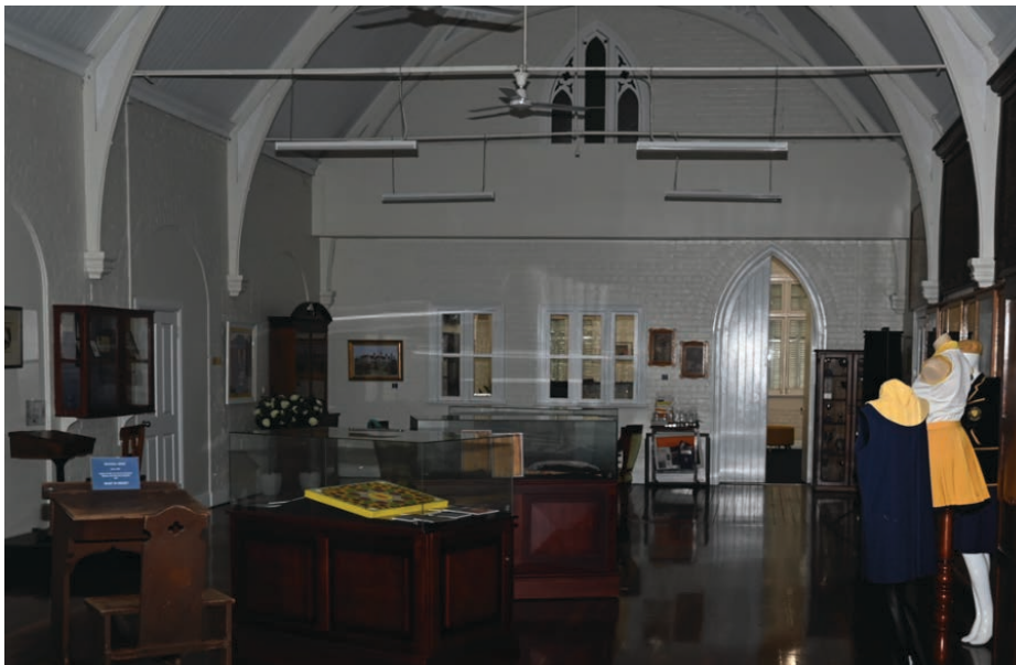
Photograph 11 Original building of brick, timber, and introduced materials.
