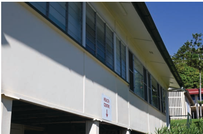
Photograph 4 Entry via western end of building
