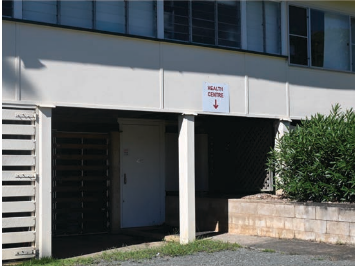
Photograph 3 Original entry was ground floor
