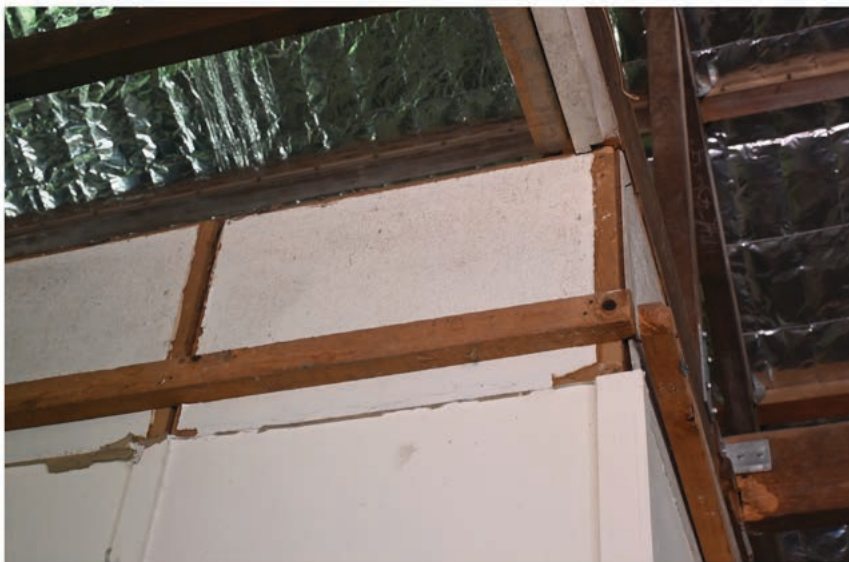
Photograph 7 Panels and infill panels removed at various locations
