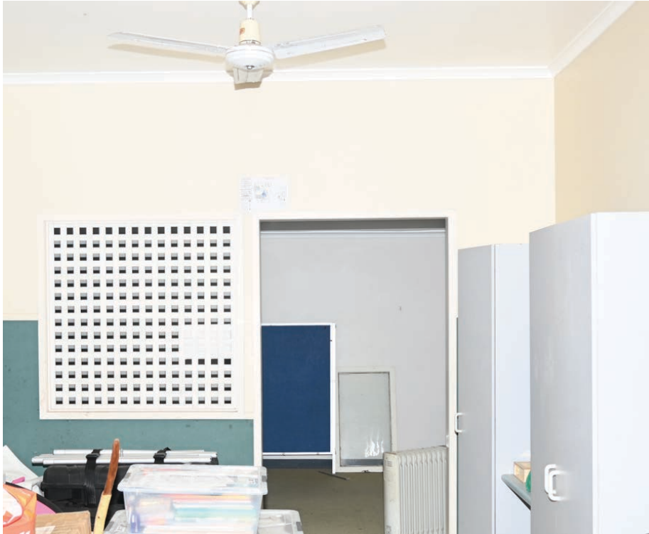
Photograph 10 Renovated office and storage areas on level one
