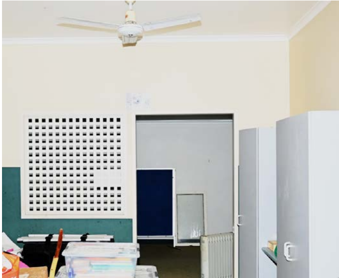
Photograph 5 Renovated office and storage areas on level one of Paterson House
