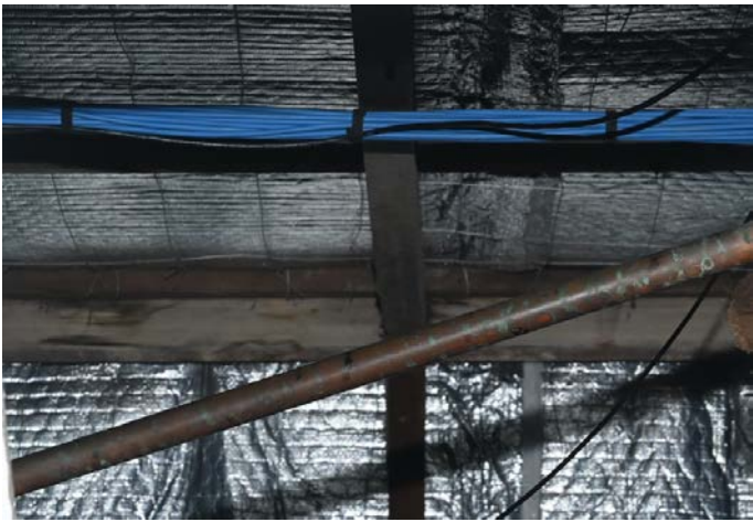
Photograph 4 Inspection of ceiling voids of Paterson House
