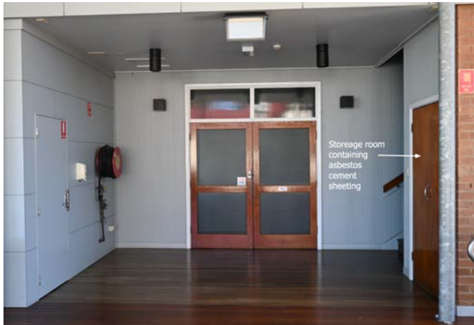
Photograph 9 Location of ACMs within McKeague Hall storage room
