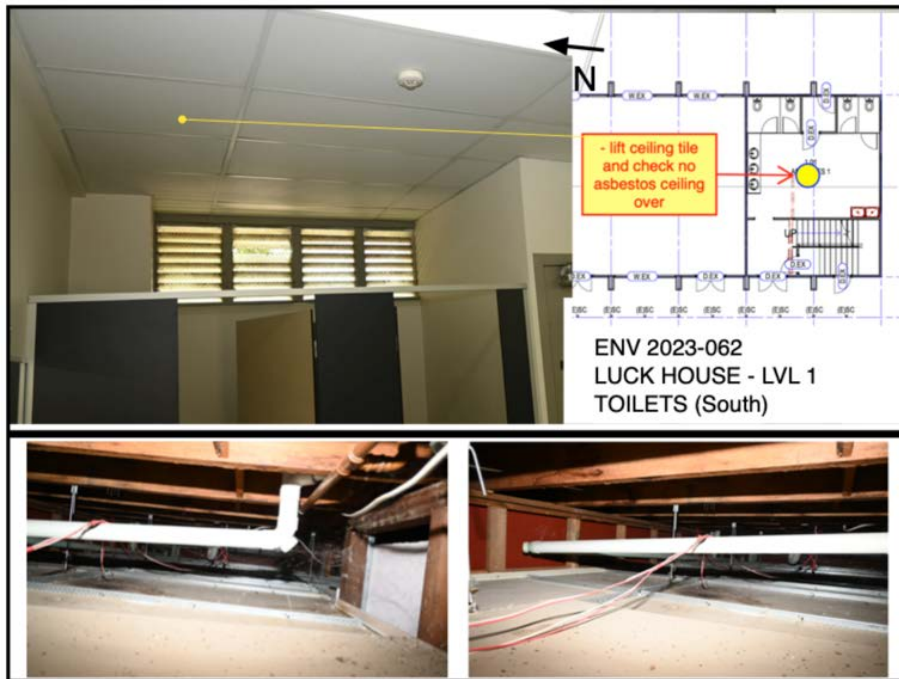
Photograph 3 Inspection of ceiling voids of Luck House
