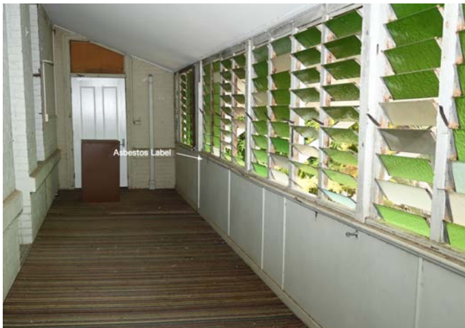
Photograph 6 A/C Wall Sheeting - Level 1 Eastern Elevation of Paterson House
