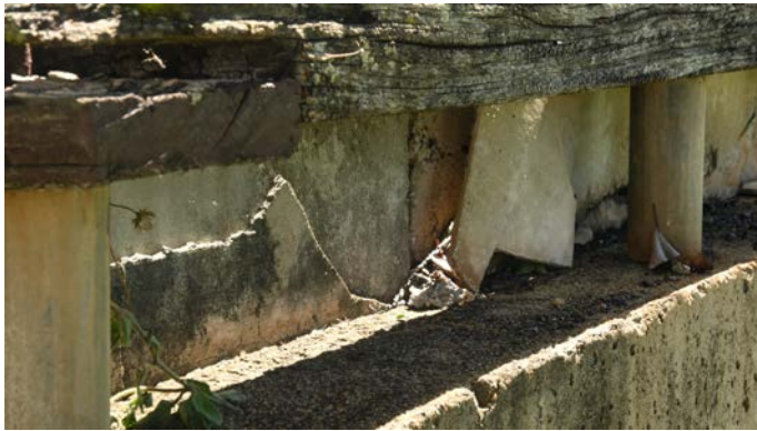
Photo 3 Form-work - Main Car Park
