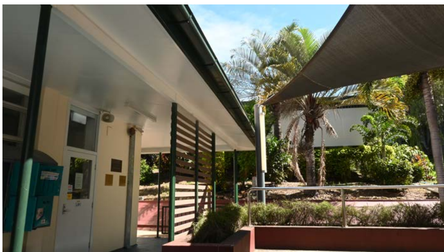
Photograph 1 Modern renovations of external ground floor areas of Jackson House
