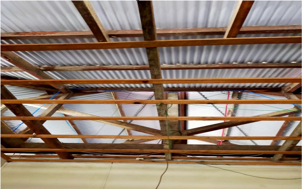
Photo: 5 Post removal of asbestos ceiling sheets.
