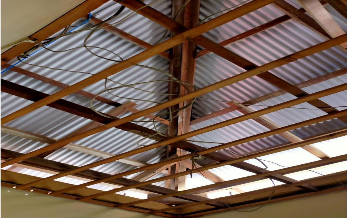
Photo: 5 Post removal of asbestos ceiling sheets.
