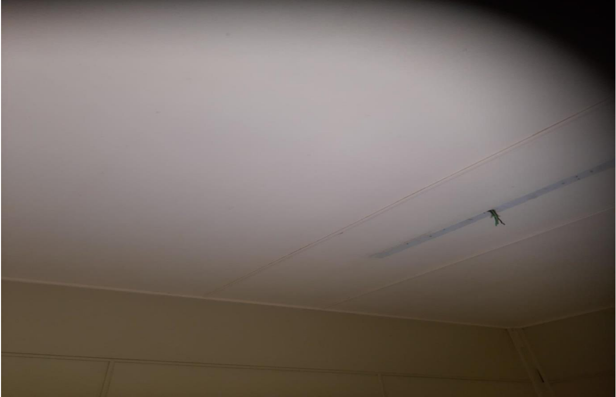
Photo: 3 Pre removal of asbestos ceiling sheets.
