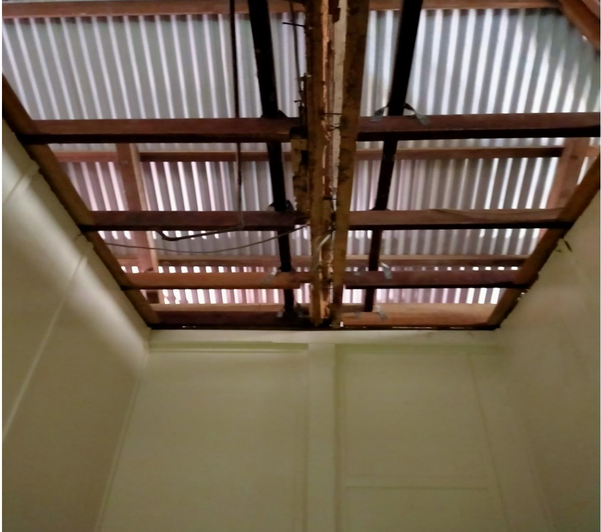
Photo: 6 Post removal of asbestos ceiling sheets.
