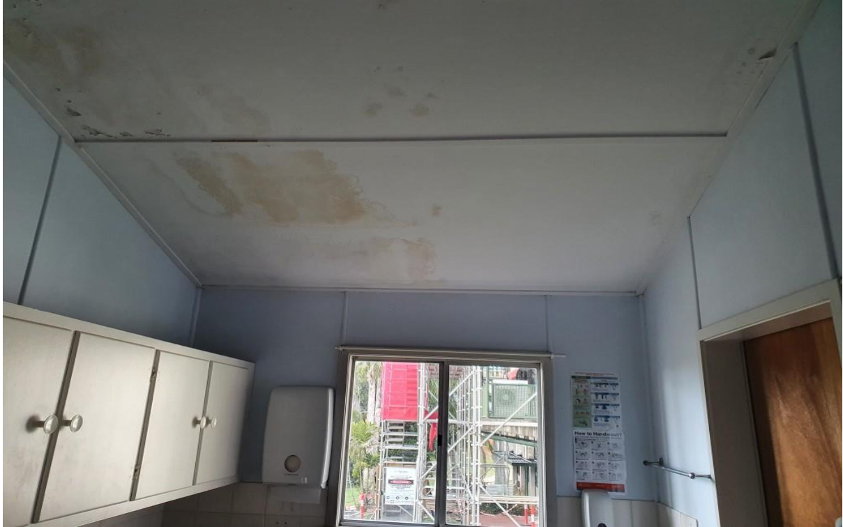
Photo:2:Pre removal of two ceiling sheets & wall sheet to kitchen central south
