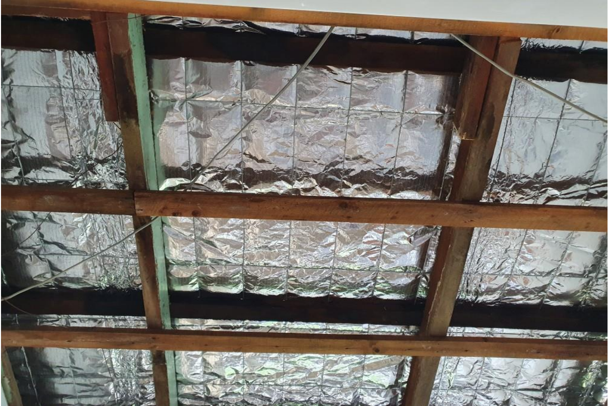
Photo:4: Post removal of two ceiling sheets & wall sheet to kitchen central south
