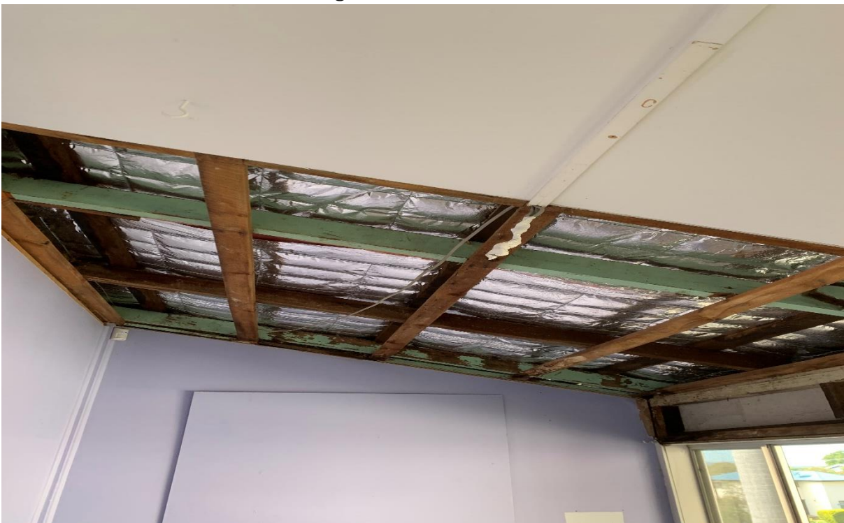
Photo:4: Post removal of two ceiling sheets & wall sheet to kitchen central south
