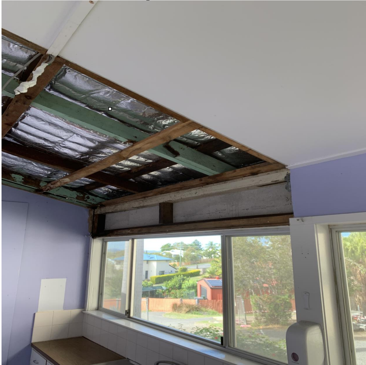
Photo:5: Post removal of two ceiling sheets & wall sheet to kitchen central south
