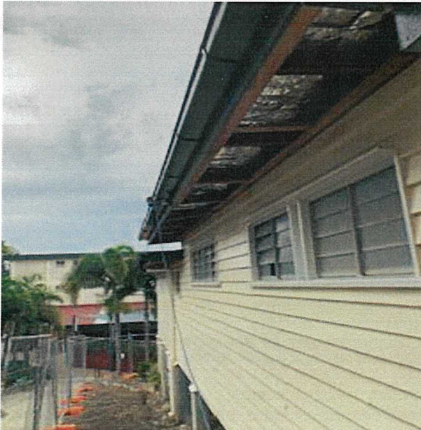
Photo ;2: Post removal soffits sheets
