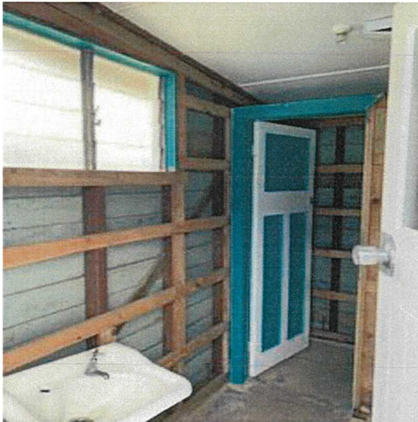
Photo :4: Post removal of wall sheets to toilet.
