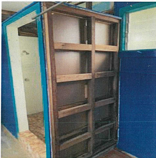
Photo :6: Post removal of wall sheets to shower
