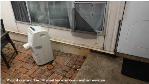
Photo 4 - cement fibre infill sheet below window - southern elevation
