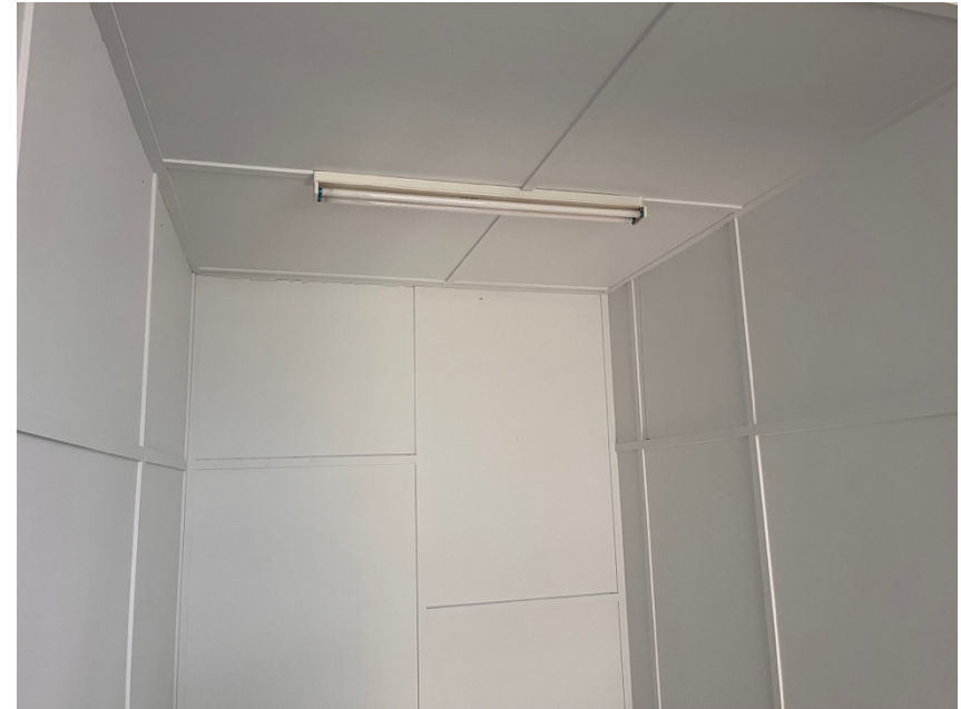
Asbestos cement ceiling sheeting – stairwell southern end of building
