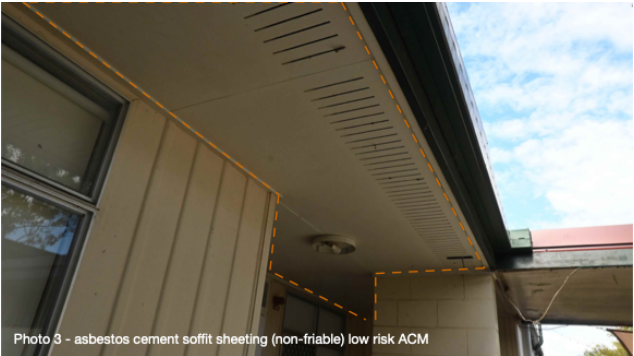
Photo 3 - asbestos cement soffit sheeting (non-friable) low risk ACM
