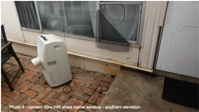
Photo 4 - cement fibre infill sheet below window - southern elevation
