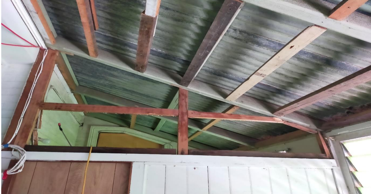
Photo: 5 Post- removal of Asbestos wall sheeting upper
