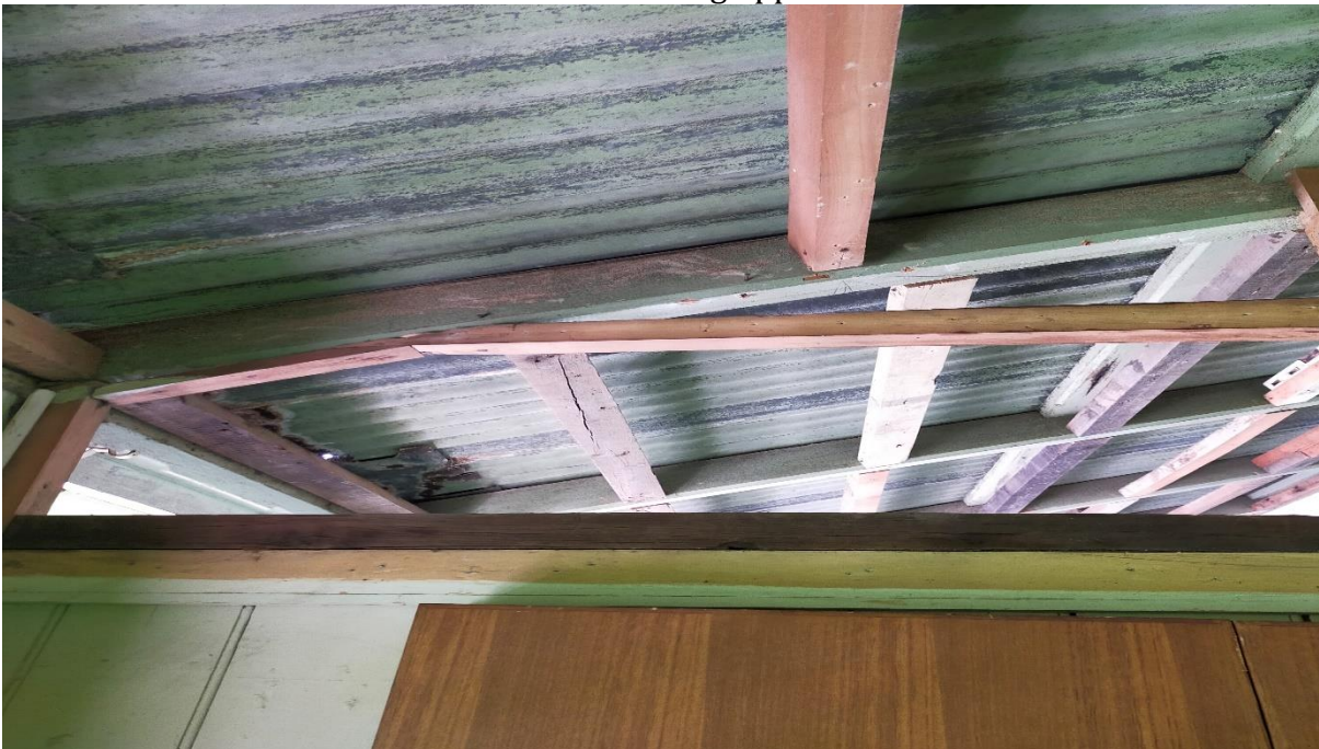
Photo: 4 Post- removal of Asbestos wall sheeting upper
