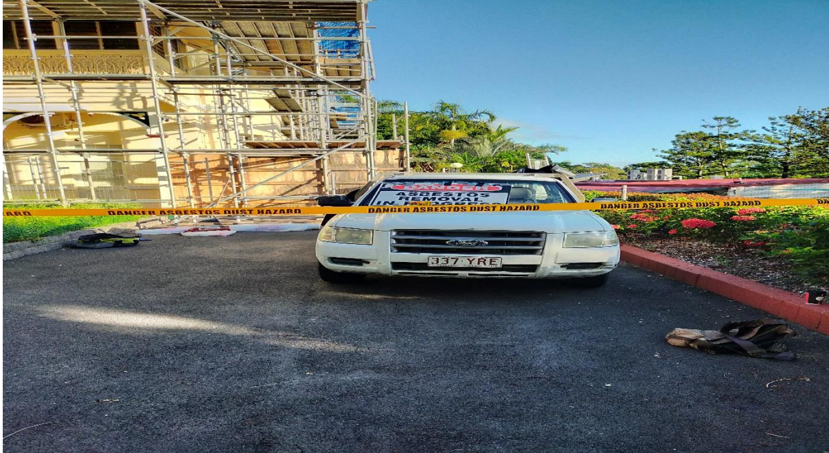
Photo: 2 Pre-removal of Asbestos wall sheeting upper
