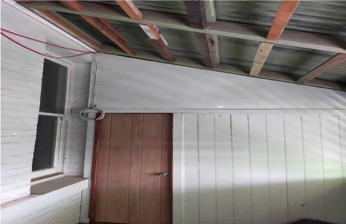
Photo: 4 Post- removal of Asbestos wall sheeting upper
