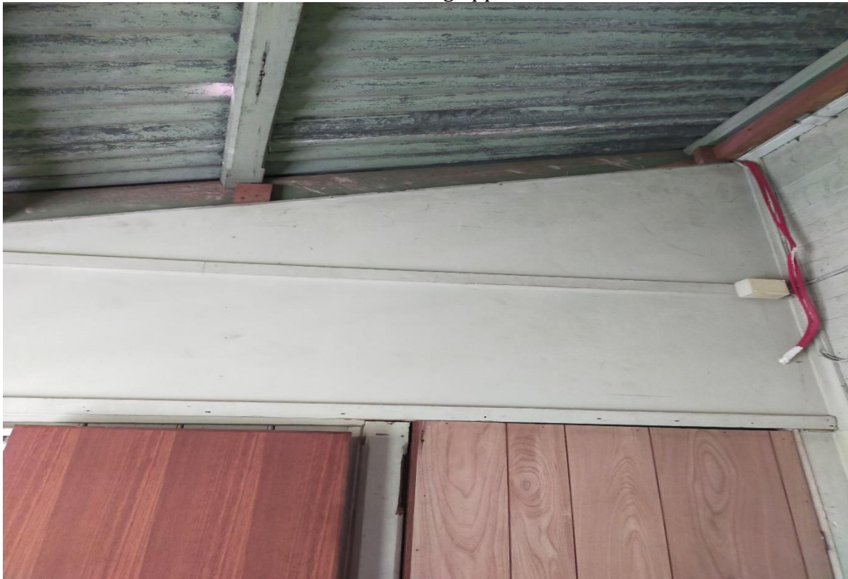
Photo: 2 Pre-removal of Asbestos wall sheeting upper
