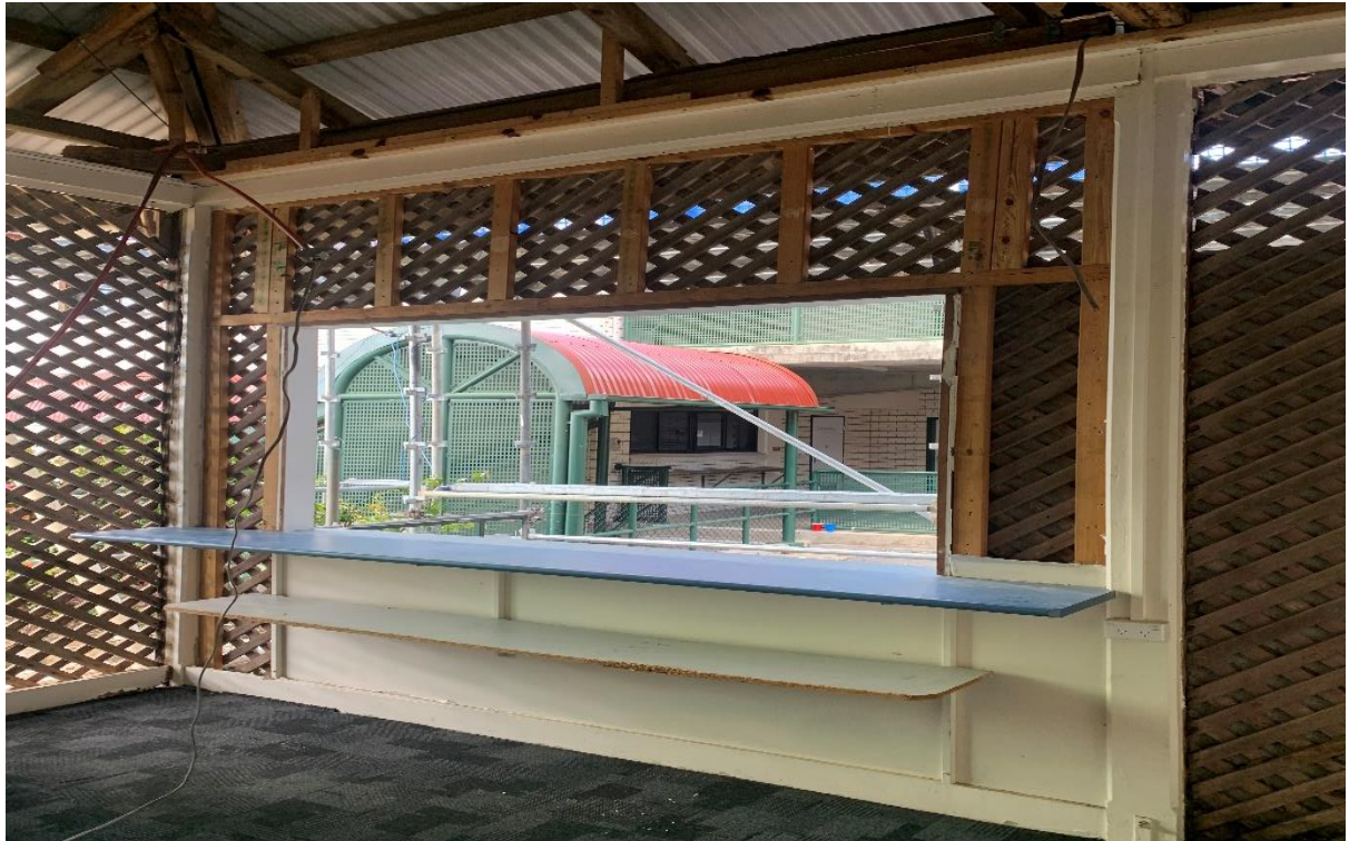
Photo: 4 Post- Removal of wall sheets around roller door
