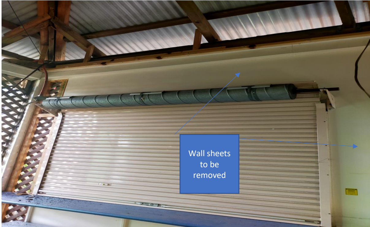
Photo: 2 Pre- Removal of wall sheets around roller door
